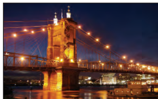
The John A. Roebling Suspension Bridge is a landmark in Northern KY and spans the Ohio River between Cincinnati, Ohio and Covington, KY. When the first pedestrians crossed on December 1, 1866, it was the longest suspension bridge in the world at 1,057 feet (322 m) main span. Today, many pedestrians use the bridge to get between the arenas in Cincinnati (Paul Brown Stadium, Great American Ball Park, and U.S. Bank Arena) and the hotels, restaurants, and parking lots in Northern Kentucky.
